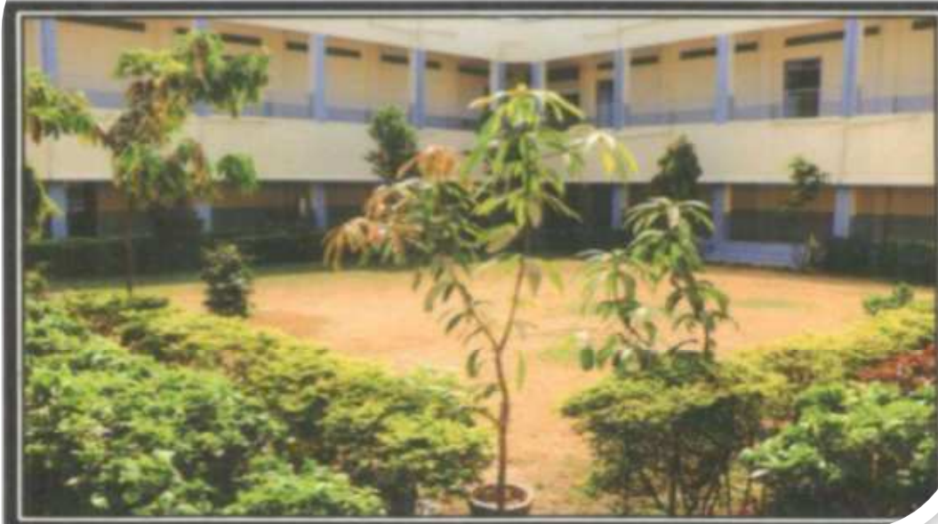
BUILDING INNER VIEW -2
