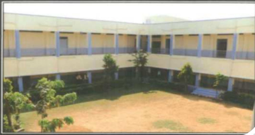
BUILDING INNER VIEW -1
